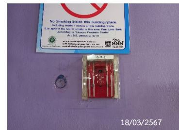
Fire Alarm Manual Station
