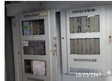
Fire Alarm Control Panel
